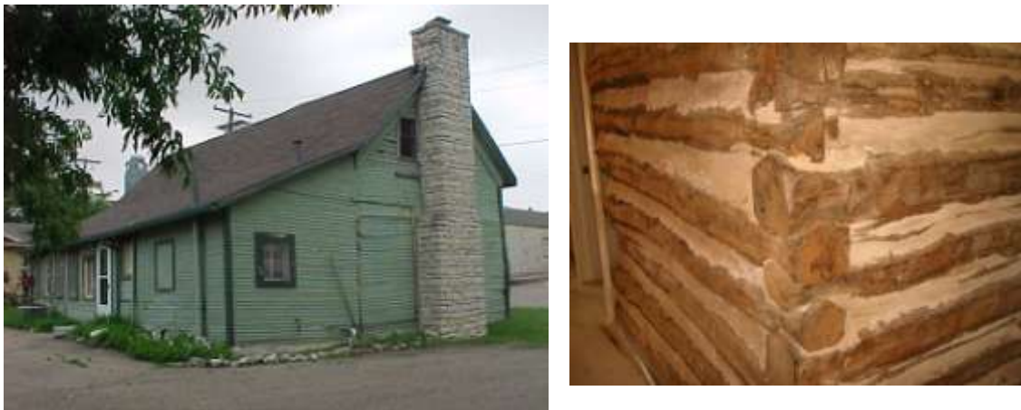
Figure 9. Austin Yeats, an Early Settler from Tennessee, Built a Log Cabin Along Lambert Branch in 1858 that Features V-Notching. As Granbury Grew, the House Developed into a Dogtrot House with a Shed Addition in the Rear. Photos by Author.
